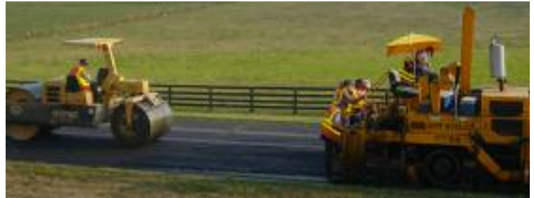
The H.G. Mays Corporation paves US 421 between Frankfort and Lexington.
