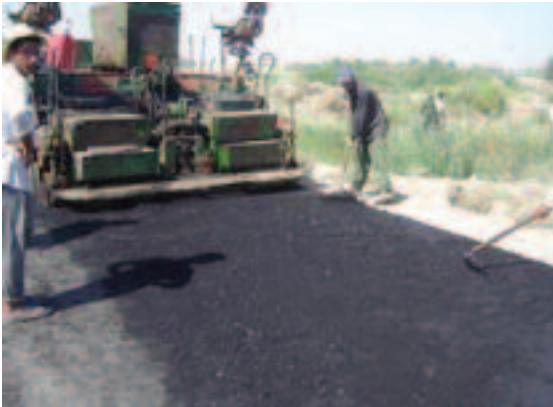
With a new paving machine on the job, work resumed
