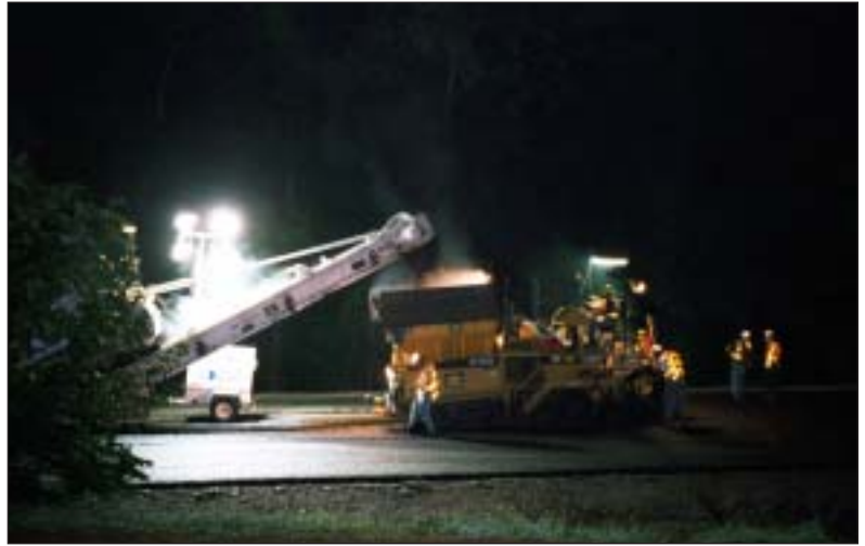
Special lighting, as seen in these photos, is required for night paving projects to provide visibility for road crews and motorists.
