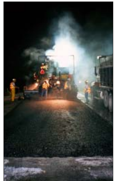
Special lighting, as seen in these photos, is required for night paving projects to provide visibility for road crews and motorists.
