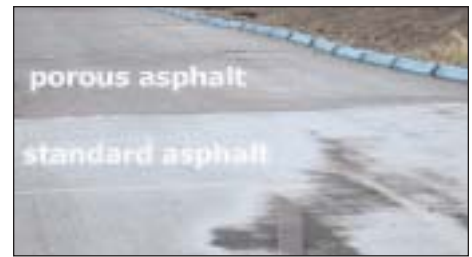
Water drains from the porous asphalt surface.
