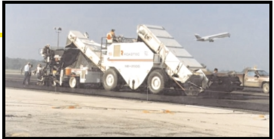
Eaton Asphalt Crews Paving at the Cincinnati-Northern, Kentucky Airport
