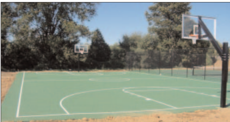
Finished basketball courts, paved with asphalt.
