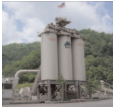
Mountain Companies Shelbiana asphalt plant in Pike County
